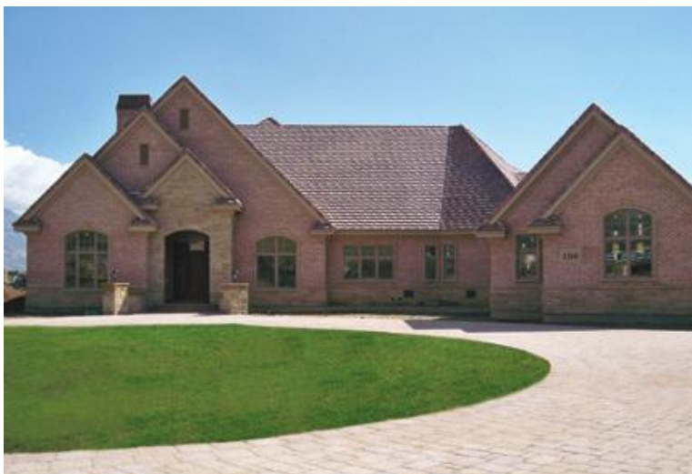
Net-Zero Residence Built With LOGIX
